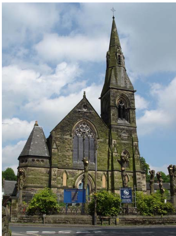
Congregational Church, Belper. Listed Grade II.
