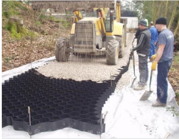
b) Application of Cellweb™ Tree Root Protection System over Vulnerable Root System
