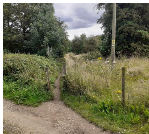
c) Cycleway Joins Blackbrook Lane at Point 2.e (View from North)
