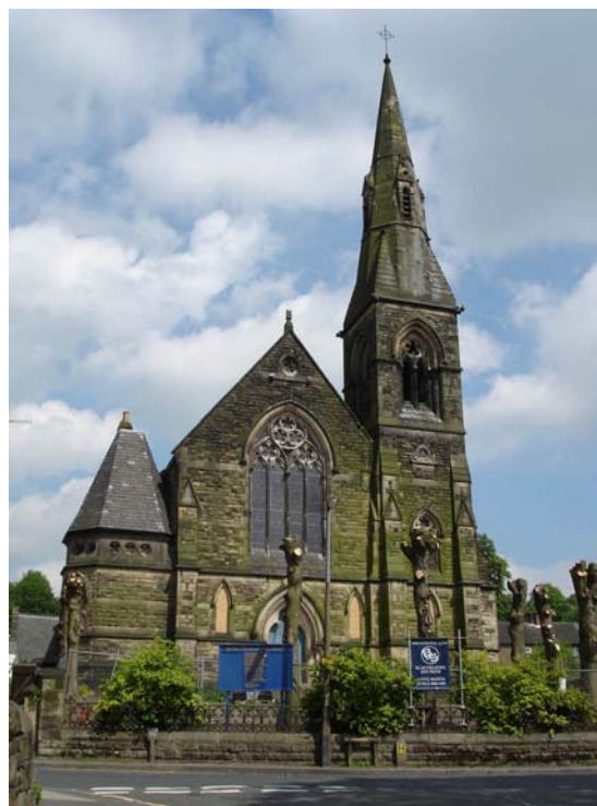
Congregational Church, Belper. Listed Grade II.
