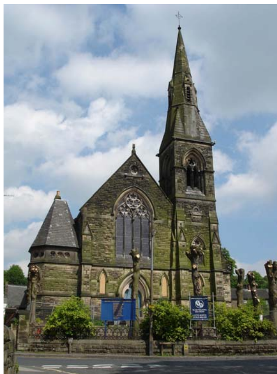
Congregational Church, Belper. Listed Grade II.
