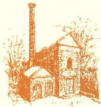
Leawood Pump House
