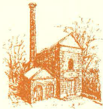
Leawood Pump House
